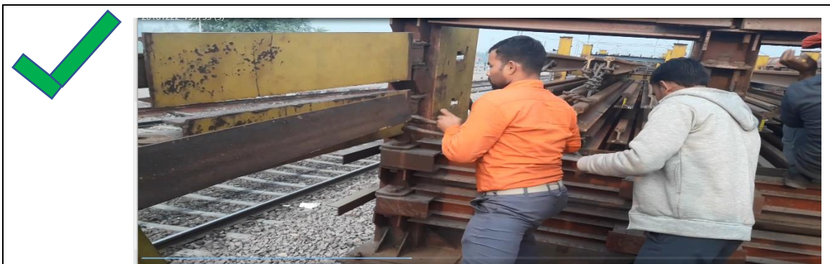
Figure 5.8: The next rail being connected after stopping the rake.
