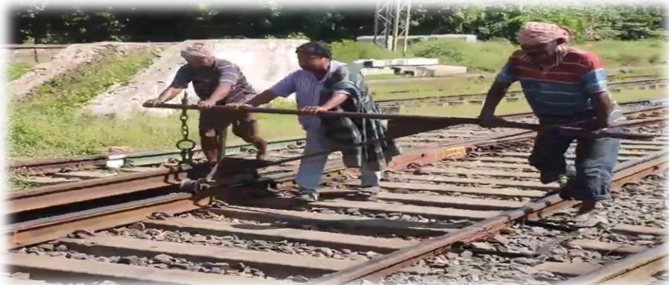
Figure 2.7 : Rail dolly for carrying rail
