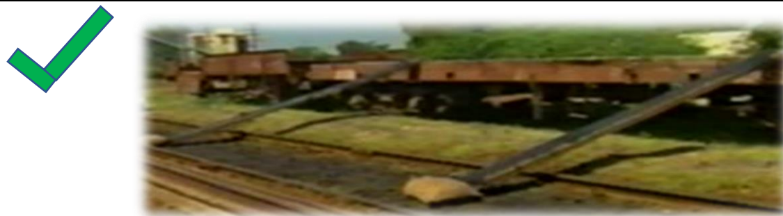
Fig 4.4 : Rail ramp for unloading of rail
