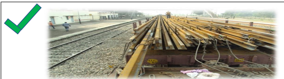
Fig 5.7: Long wire rope at unloading end of each rail.
