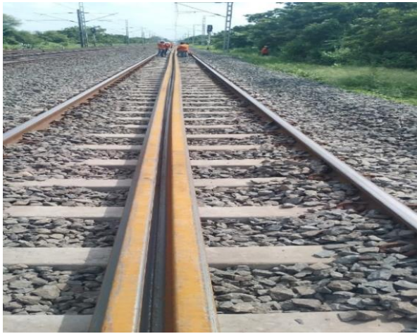
Fig 5.10: 20RP Unloaded in between running rail
