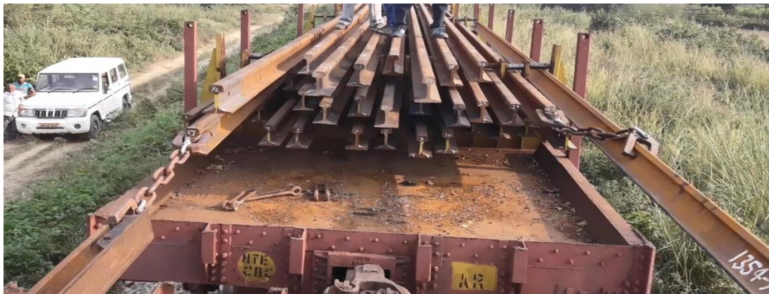
Fig A4 : Automatic linking of left rail and sliding over right rail
