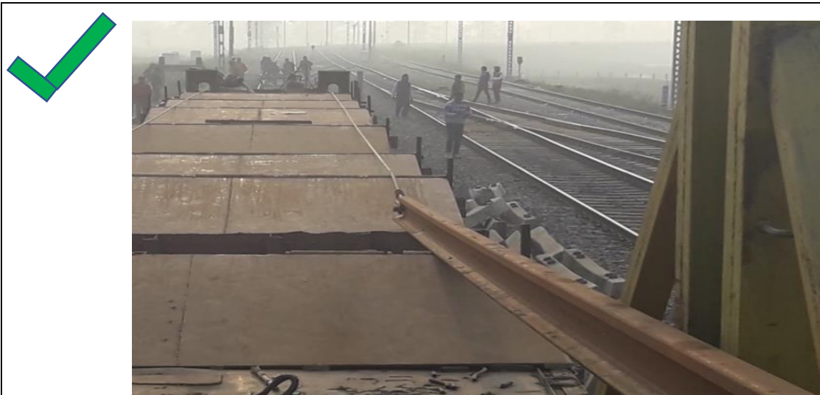
Figure 5.5: First Rail tied to track through chute
