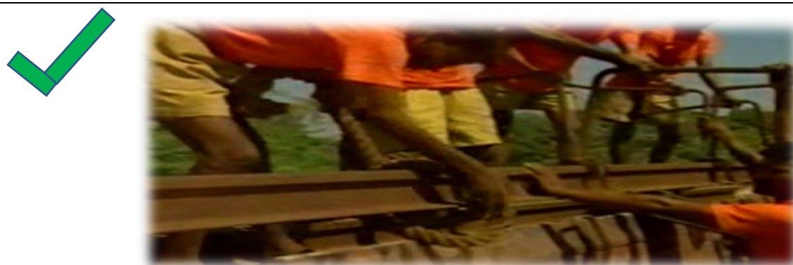
Fig 4.5: Manila rope being tied to rail being unloaded.
