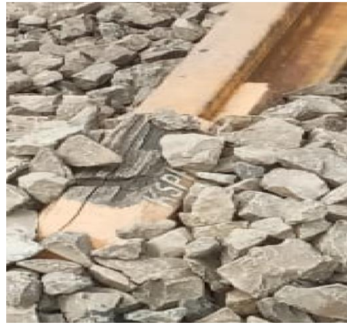
Fig 5.11: Wooden block provided at end
