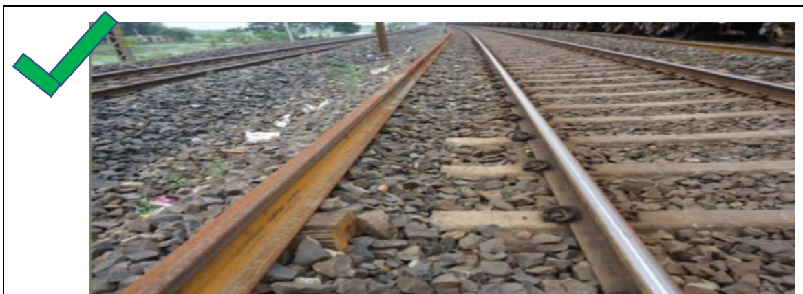
Fig 6.1: Rails supported on wooden block
